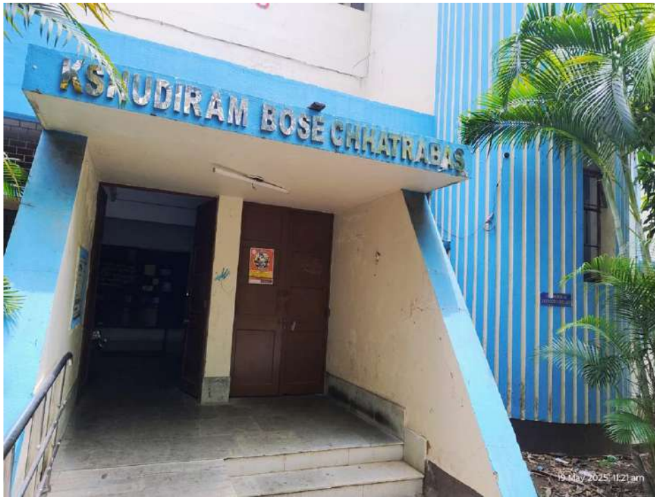
Figure 5: CCTV Camera installed at the Entrance of Boys' Hostel in the Vidyasagar University campus
